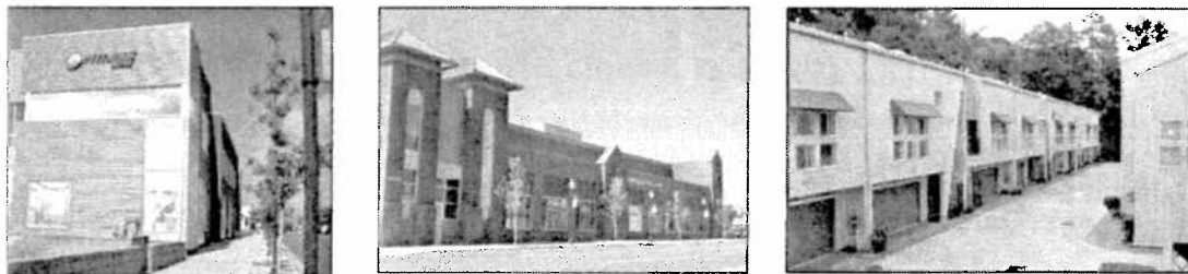
Images showing appropriate building materials within TOD Transition Character Zone.
